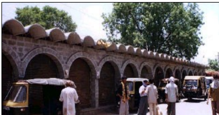
Figure 6 Building production from waste: stone-cement blocks, ferrocement channels
